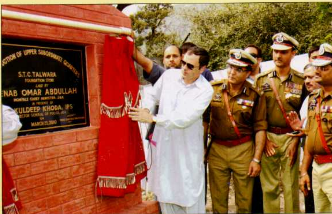
Hon'ble CM J&K laying the foundation stone for construction of upper subordinate quarters complex at STC Talwara on March 25, 2010
